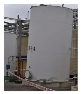
This damaged tank was damaged in the 2010, 8.8 magnitude earthquake in Chile. This tank looks to be about 10' tall and 8' in diameter. It was anchored, and the liquid in the tank sloshed causing the structural damage. We do not know if the tank was designed for this type of seismic loading.
