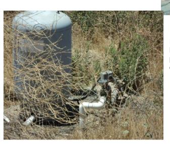
Here is an example of a well that will have major failure during a wildfire. The plastic piping and electrical will be damaged.
