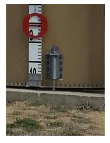
In this example, brackets are bolted to the shell of a steel water storage tank, and attached with a long bolt cast into the concrete.
