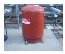
Simple angle iron clips are bolted to this pressure tank's bottom and the concrete.
